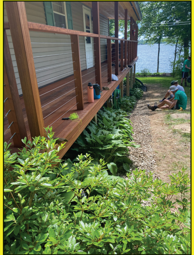
New dripline trench installed here.
